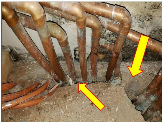
4. Piping through the concrete have holes and are badly cracked and will need to be epoxy sealed to prevent water and moisture from penetrating.
