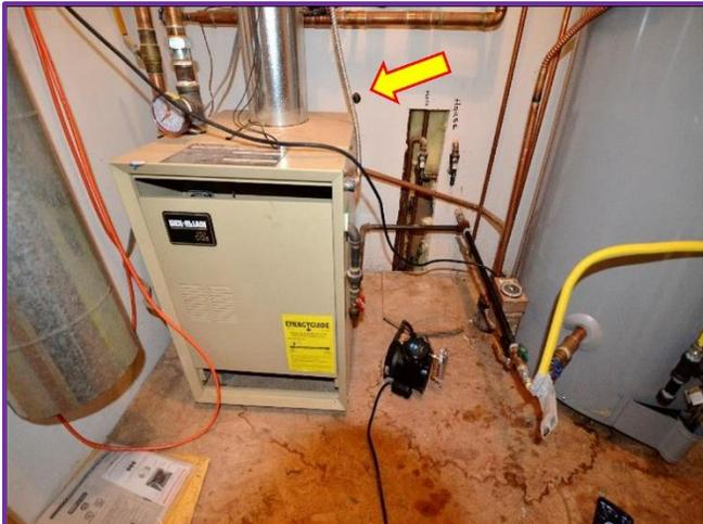
1. Mechanical closet is now the Active Mold Zone and will need immediate Remediation. Hole cut for the air test on the Mechanical and Pantry wall.
