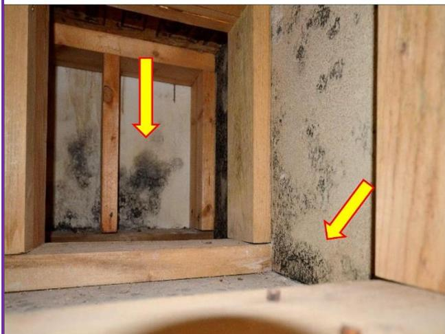
3. Black mold spots found under the Mechanical platform on the walls and sill plate; whereas the drywall will need to be removed for Remediation.
